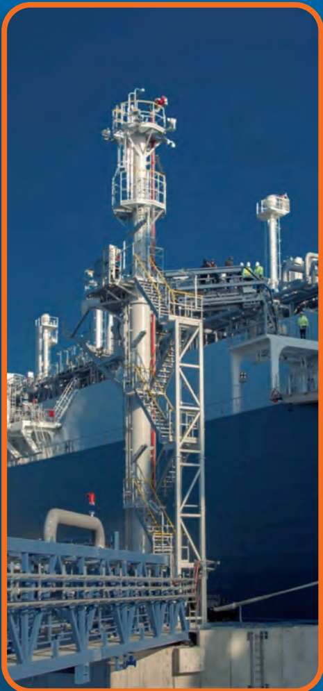
Column with fire monitor support on top. The telescopic gangway provides support for the ship-to-shore power supply. Klaipėdos – Lithuania.
