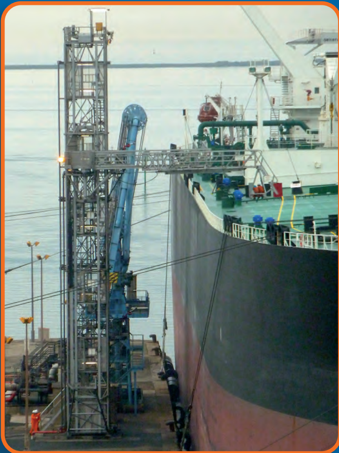
One of four gangway towers with lift platforms and telescopic gangway, with provisions for corrosive dust laden environment. Marseille – France.
